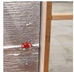
The same wall without the batt insulation has a u-value of 0.85 W/m<sup>2</sup>K. (Calculations based on BS EN ISO 6946 wall procedures). It is reasonable to acknowledge that any cavity wall arrangement with insulation gaps cannot match the thermal integrity of a cavity wall arrangement as intended.
