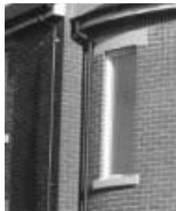
Curved lintel and curved masonry protected by cavitytray of equal radius.
