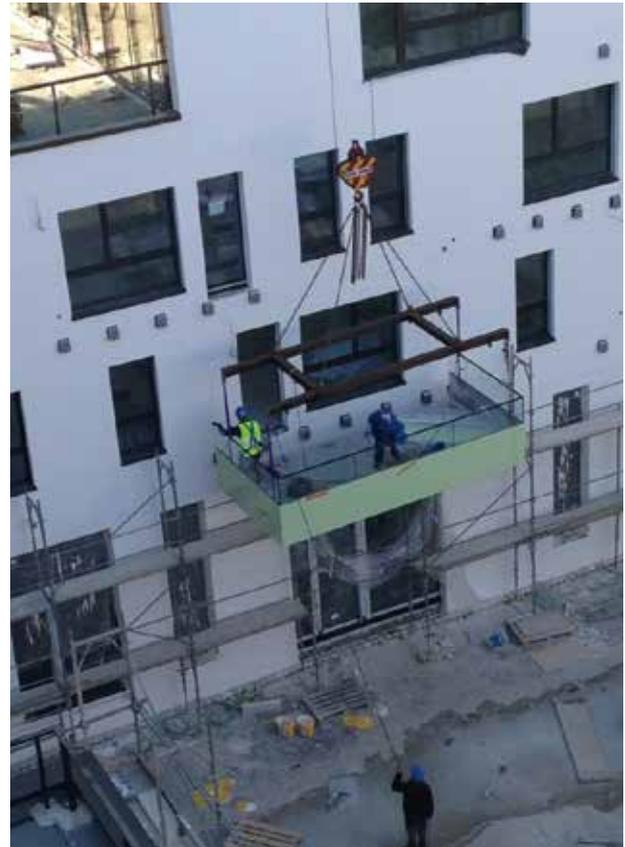
The metalworker completely prefabricated the balconies, based on the architects' plans, using sheet aluminium, Mineralit, stainless steel and laminated safety glass. The balconies were lifted into place by a crane fitted with special lifting gear.
