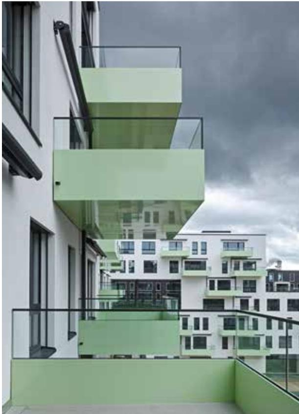
The Schöck Isokorb® elements, a total of 300 – between four and six per balcony, depending on size – were installed while the structure was being built, with some welded to the reinforcement to prevent tipping during concrete application.
