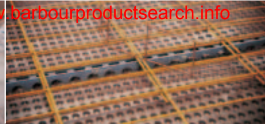
Reinforcement-mesh spacers are safely held in place.
