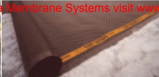
Overlaps should be 20 cm minimum.
