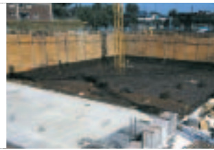
DELTA®-GEO-DRAIN Quattro protects compression-sensitive waterproofing.
