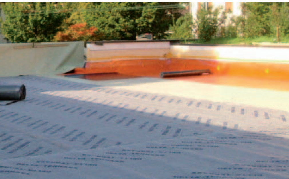
Herbaceous roof detail – connection to a double-shelled masonry structure.
