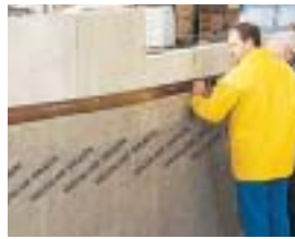
DELTA®-NP DRAIN ensures reliable drainage.
