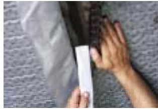
Integrated self-adhesive tape for laying precision.
