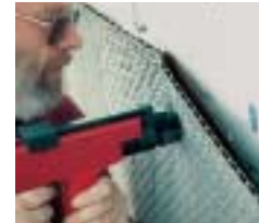
A typical way of installation is to attach the dimpled sheet with a gas or nail gun.
