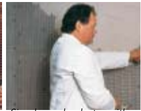
Simply apply plaster with a trowel.
