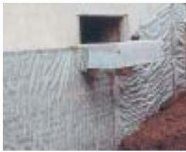
DELTA®-DRAIN keeps foundation walls dry and provides extra heat insulation.
