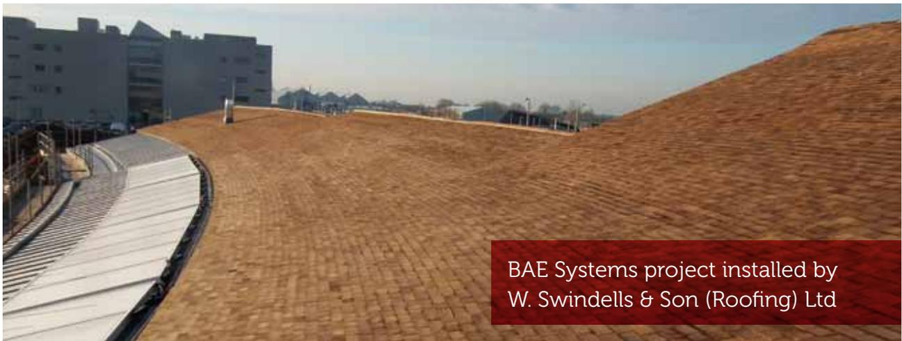
This 2,500m<sup>2</sup> building, with an elongated curve and consisting of over 80,000 individual shingles, would have been impractical to fix by traditional hand nailing. The staple fixing method has proved to be a very practical and cost effective method of fixing shingles.
