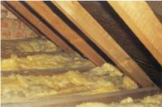
Mineral fibre loft insulation blocking eaves ventilation
