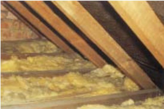
Mineral fibre loft insulation blocking eaves ventilation
