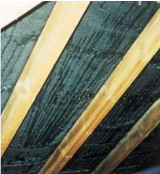
Condensation occurring on the underside of sarking felt
