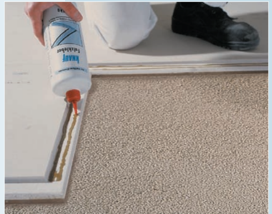
Applying Brio Joint Adhesive to the edge
