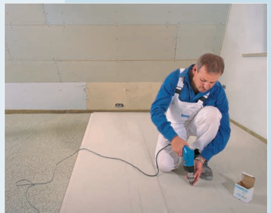
The glued boards are quickly screwed together
