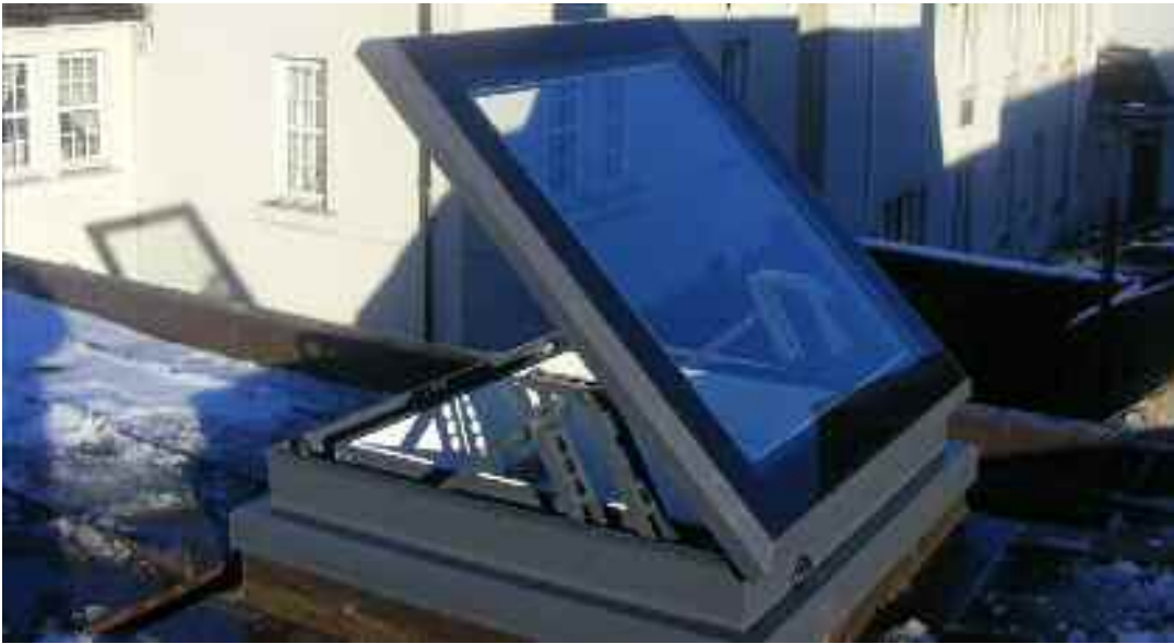
X-Vent Rooflight (AOV) Smoke Vent
