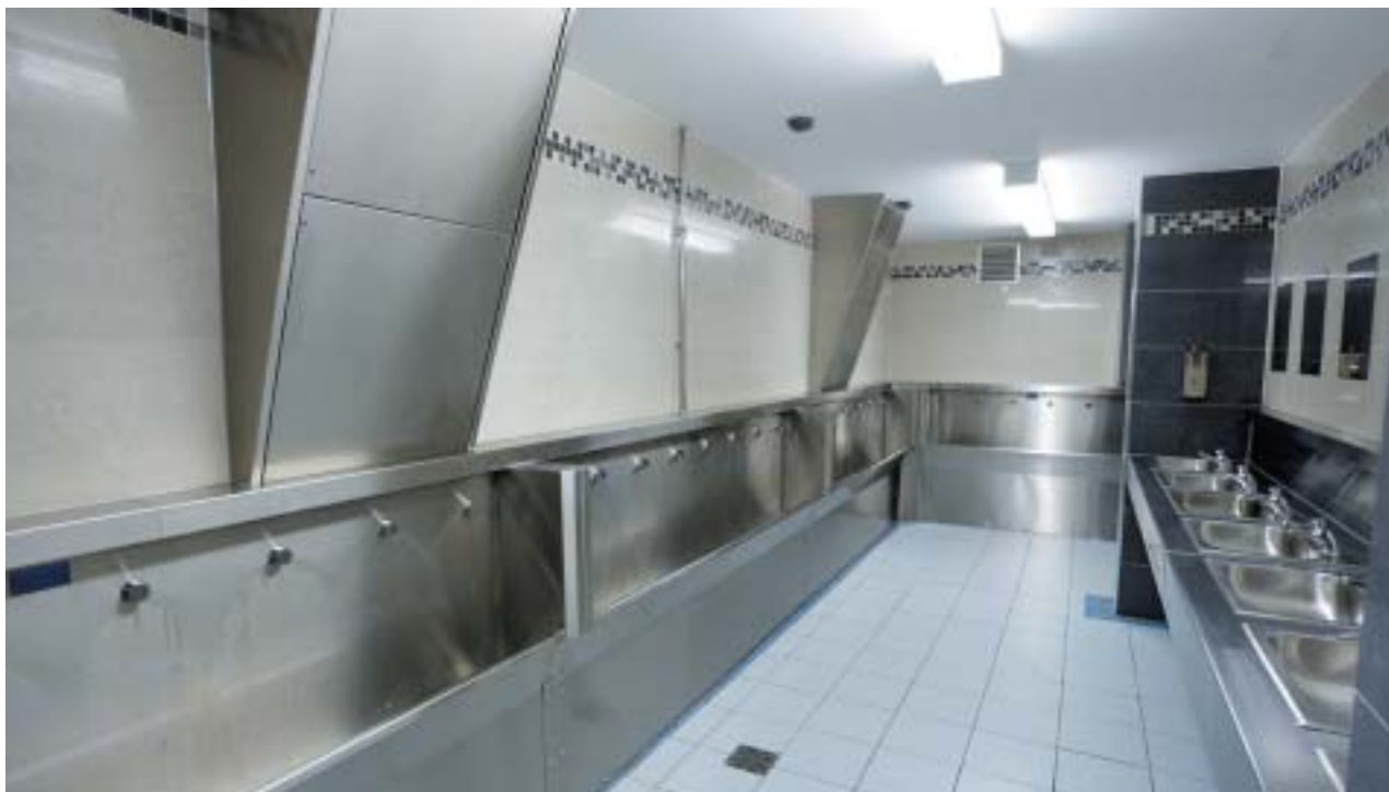
Stainless steel wall-hung trough urinal complete with anti-vandal undershield and stainless steel boxing to services.
