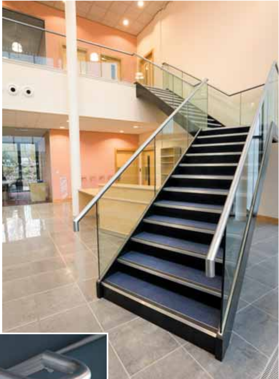
Staircase complete with structural glass balustrading, stainless steel top rail. Project: Pendragon, Nottingham.
