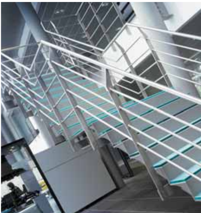
Glass treads complement this staircase in a prestigious car showroom.
