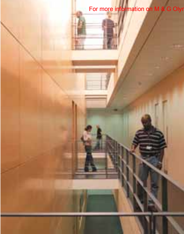
Flat bar balustrade.
