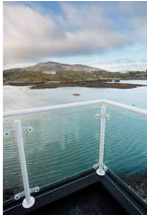
Polyester powder coated balcony balustrade with glass infill.
