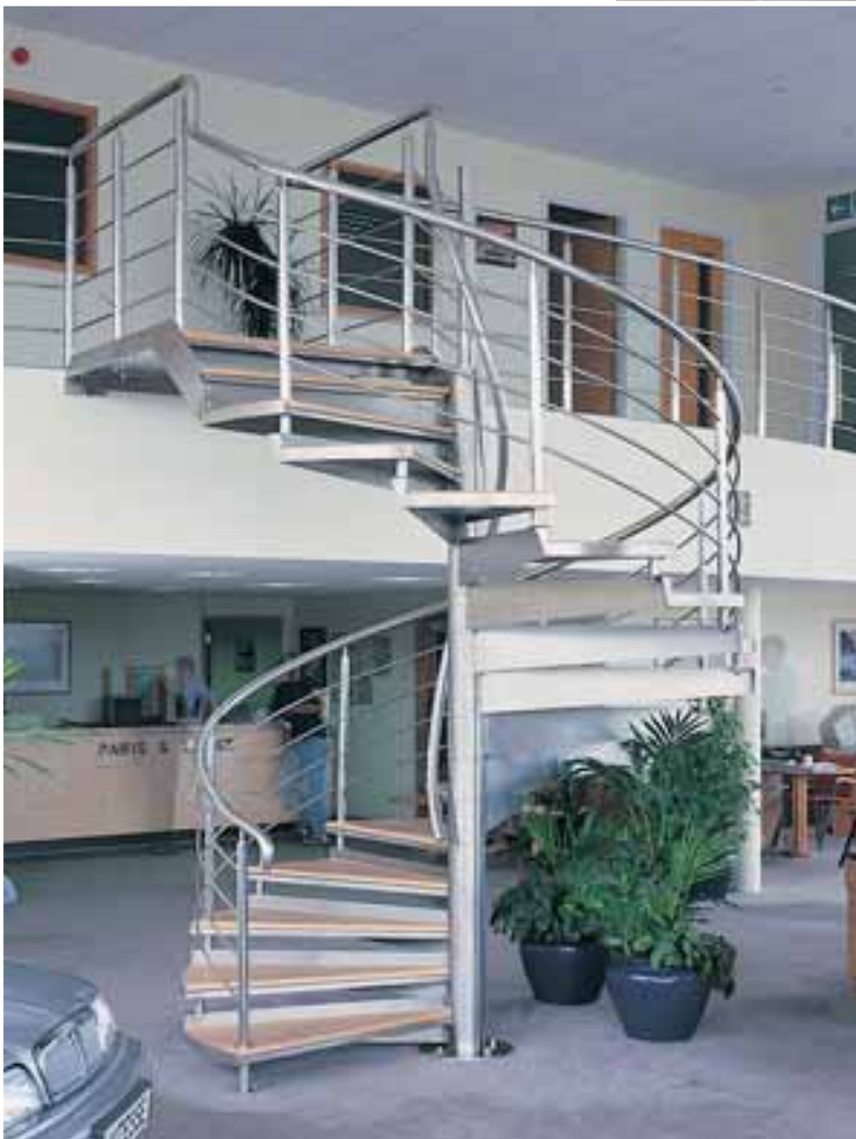
Stainless steel spiral staircases and balustrade with rod infills.
