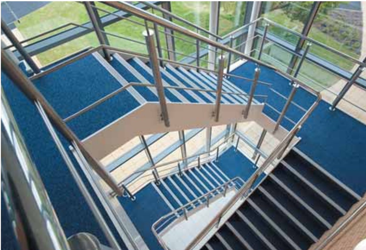
Staircase complete with stainless steel balustrading.
