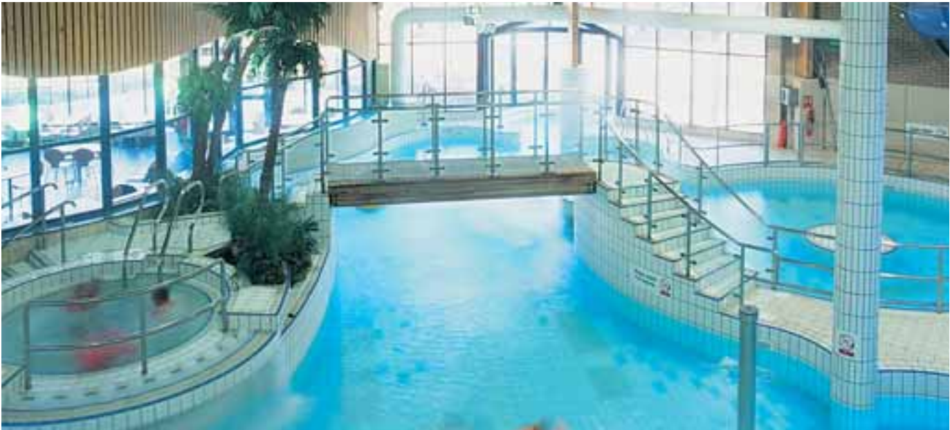
Stainless steel balustrading complete with toughened glass panels. Stainless steel twin rail barriers and spa pool access ladders.
