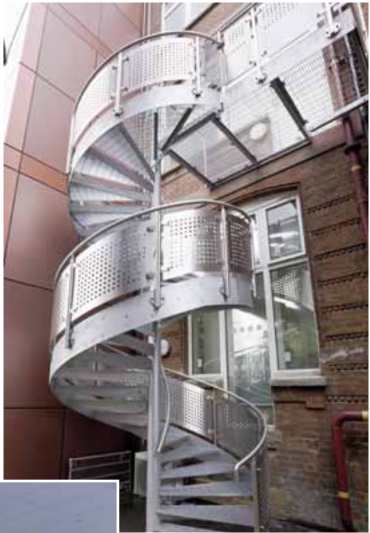
External mild steel spiral fire escape stair with perforated aluminium panel infills.
