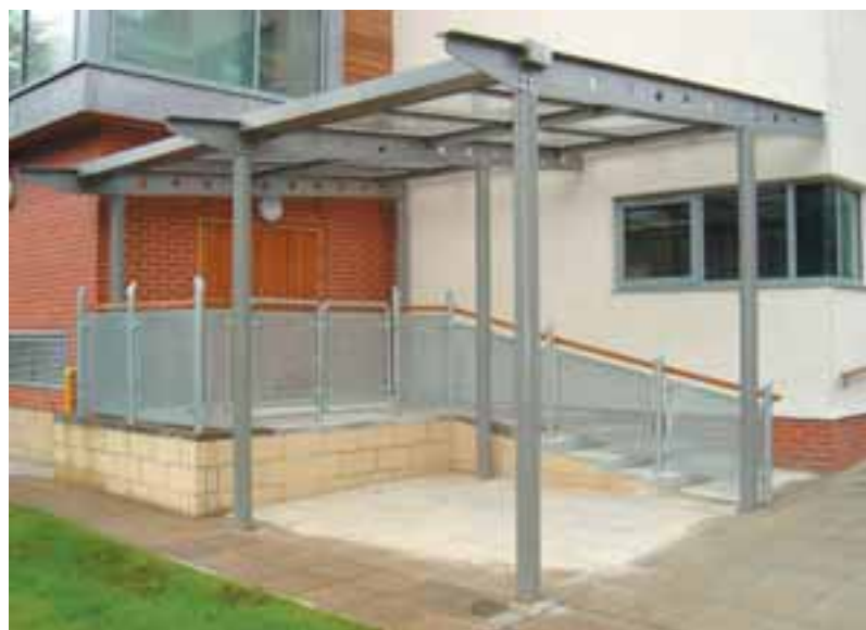
Canopy and galvanised external balustrading with a timber top rail and mesh infill panels.
