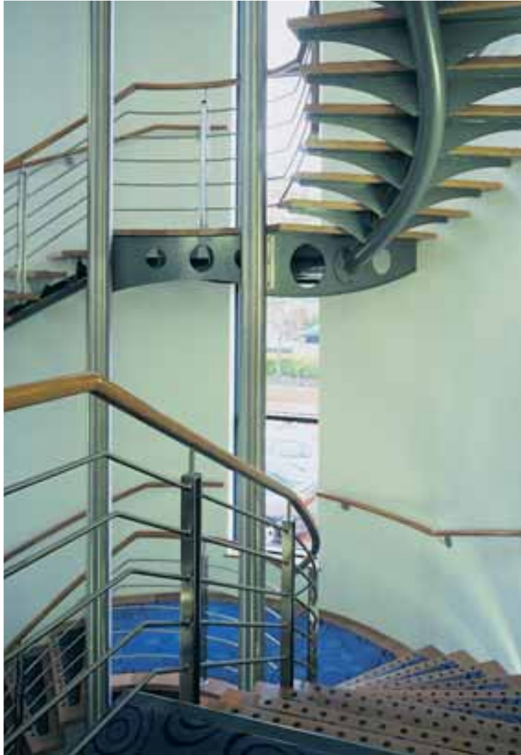
Mild steel polyester powder coated helical staircase and stainless steel balustrading complete with stainless steel support columns, timber treads and top rail. Situated in the prestigious offices of a surgical instruments manufacturer.
