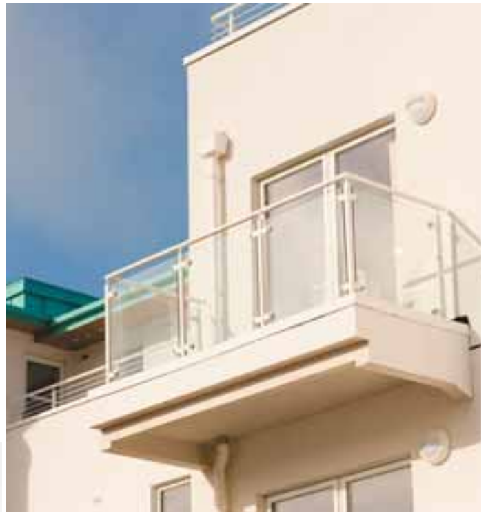
Polyester powder coated glass infill balcony balustrading to luxury apartments, Holyhead Marina.
