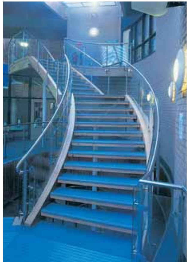
Stainless steel curved balustrading with curved toughened glass infills complete this staircase perfectly at The Quays Swimming & Diving Centre in Southampton.
