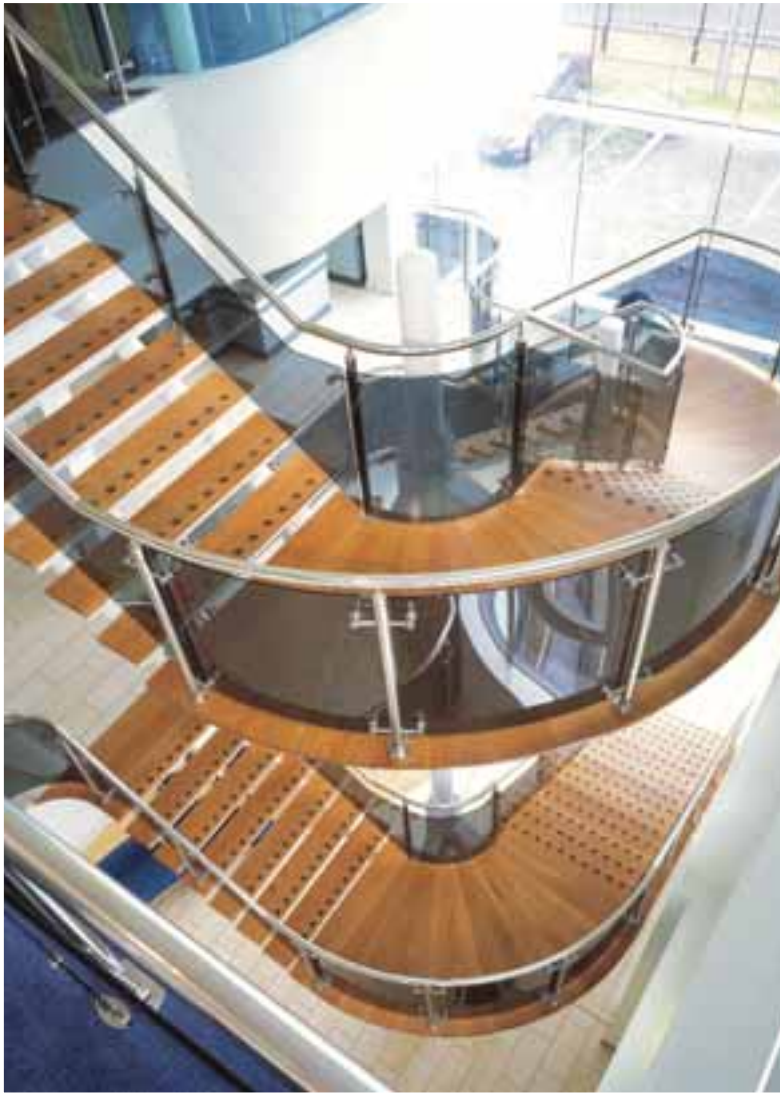
Curved glass complements the balustrading on this feature staircase at Searchlight Electric in Manchester.
