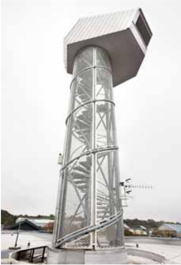
Self-Coloured Perforated Aluminium Cladding Panels To Observation Tower, The Tank Museum, Bovington.
