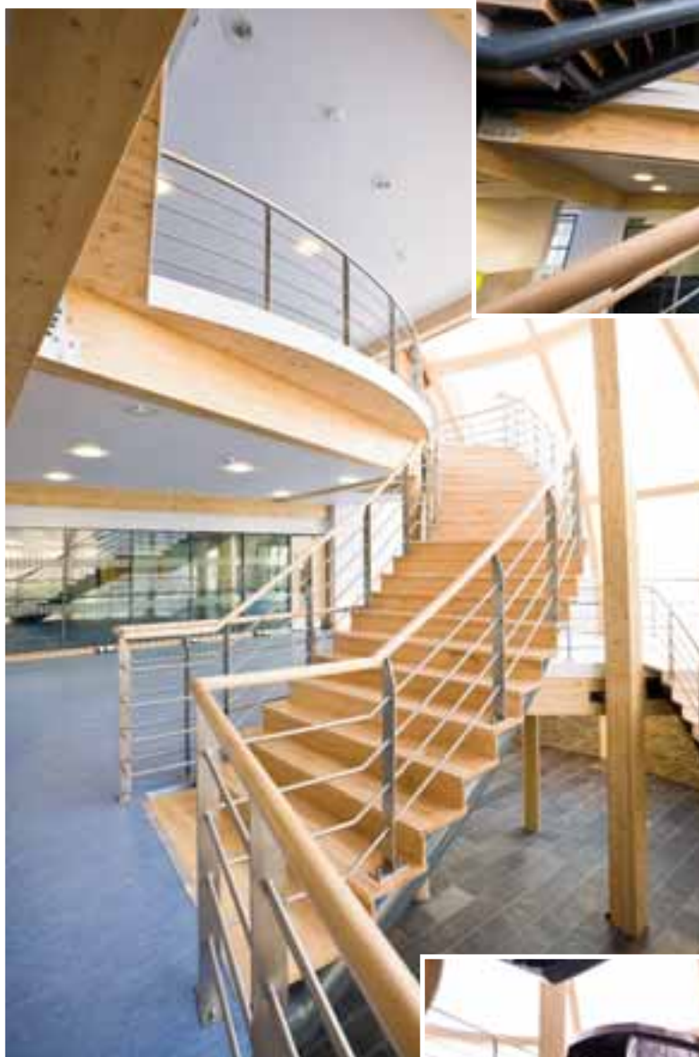
Site: the William Smith Building: a newbuild 4-storey sustainable office facility for the British Geological Survey, Keyworth. Two helical staircases complete with tubular stringers, landings, timber treads and risers, stainless steel balustrading and timber handrail.
