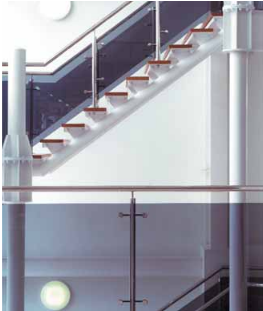
Staircase with spine stringers.
