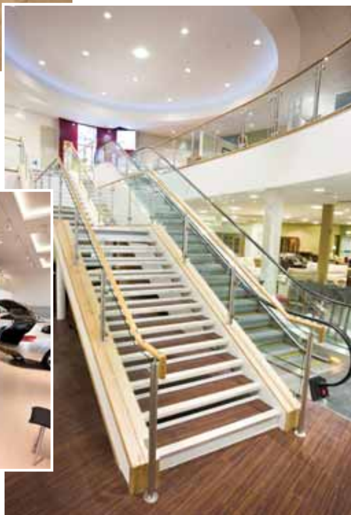
Feature stair complete with glass infilled stainless steel balustrade, solid oak capping and top rail
