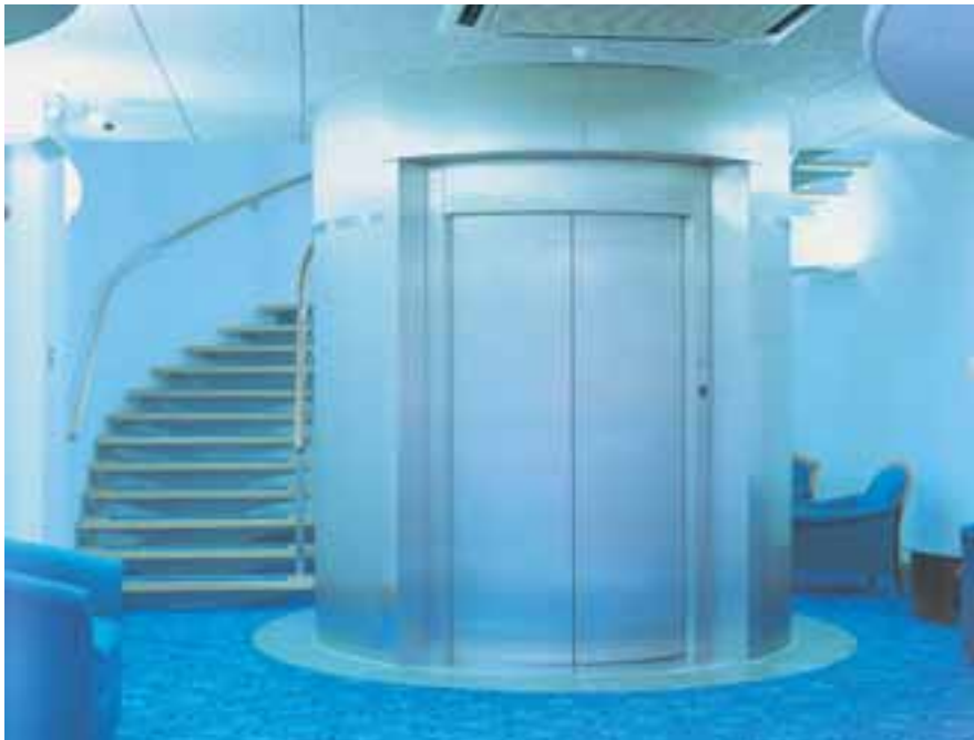
Stainless steel lift shaft cladding.
