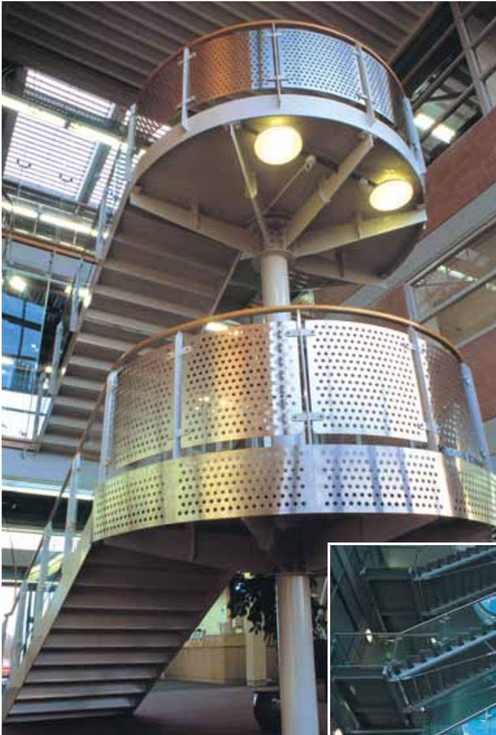
Mild steel staircase landings, support column complete with glass and stainless steel perforated sheet infilled balustrading and timber top rail.
