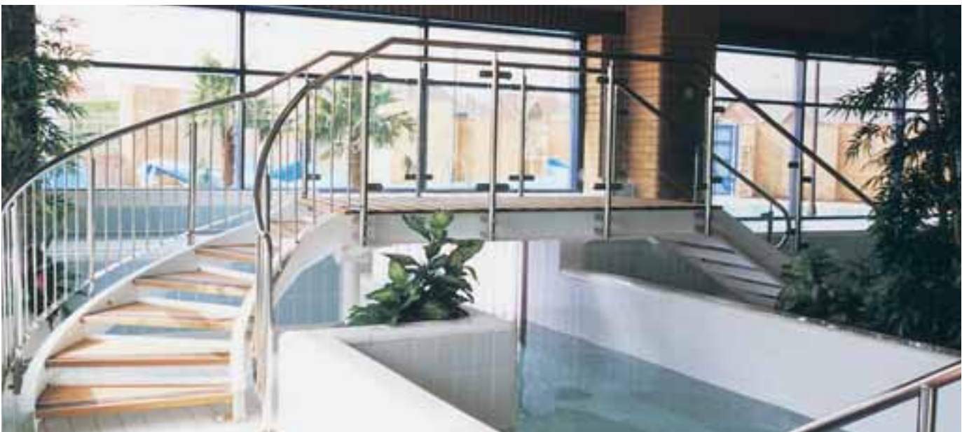
Mild steel bridge, stainless steel balustrading complete with toughened glass and stainless rod infills. Designed by M & G Olympic Products Design & Development Department.
