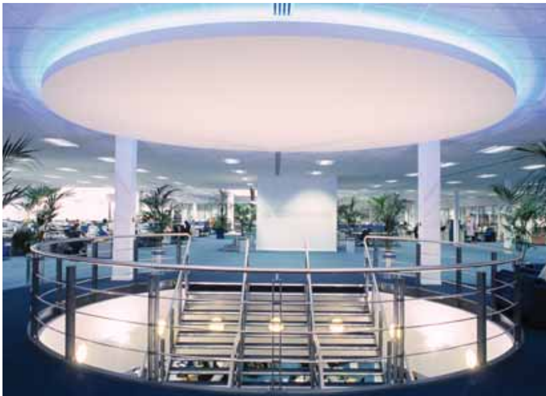
Mild steel polyester coated balusters complete with stainless steel rod infills and top rail.
