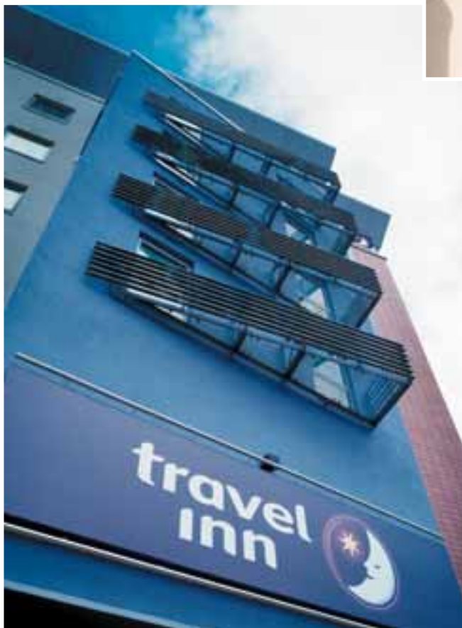
Decorative, galvanised balconies.
