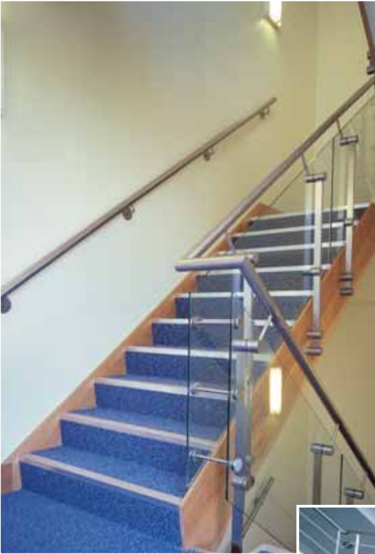
Mild steel staircase clad in timber (by others) complete with glass infilled balustrade.
