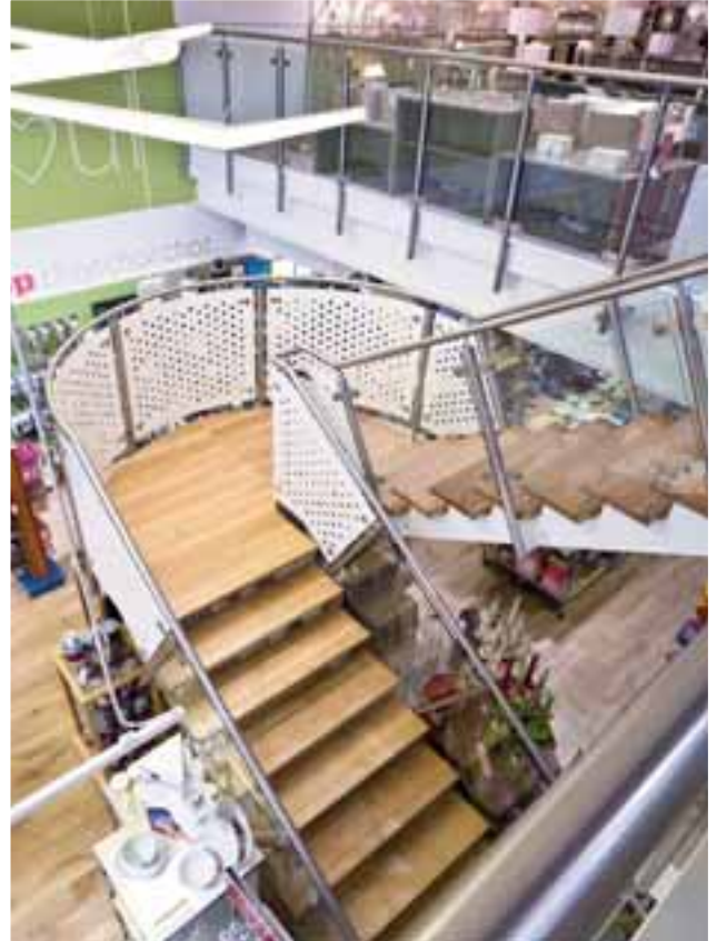
Feature stair complete with timber treads & half landing, complete with glass infills & polyester powder coated perforated infills.
