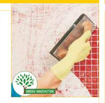
Super fine, high performance cementitious grout for joints up to 4 mm.
