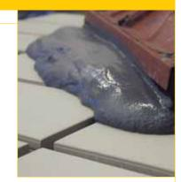
High performance cementitious mortar, for grouting joints of 4 to 20 mm in stone or ceramic industrial floors which are subject to considerable loads.
