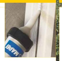
One component, thixotropic, rapidhardening polyurethane sealant and adhesive with a high modulus of elasticity for joints subject to movements up to 20%.
