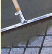
Pozzolanic, fast-setting mortar with very low water absorption and high mechanical strength for grouting paved floors with joints from 5 to 30 mm subject to heavy stresses and intense traffic.
