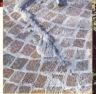
Three-component, epoxy drainage mortar for grouting paved floors with joints at least 5 mm wide subject to medium-intensity stresses.
