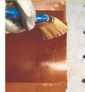
One-component, solvent-free primer for non-absorbent surfaces.
