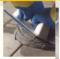
Two-component, acid-resistant epoxy mortar which is particularly easy to apply and clean, for grouting tile joints wider than 2 mm.
