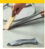
Closed cell polyethylene foam cord for the correct sizing of movement joints. Is available in skeins where the length is proportionate to the diameter.
