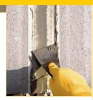
**Two-component thixotropic** polyurethane sealant for joints with maximum 10% expansion of the initial size.
