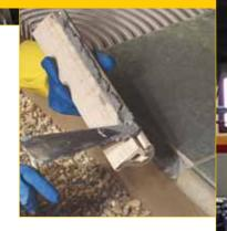
Two-component, epoxy adhesive with no vertical slip for ceramic tiles and stone material.
