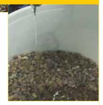
Solvent-free, one component polyurethane binder for mixing drainage mortar and grout for paved floors.
