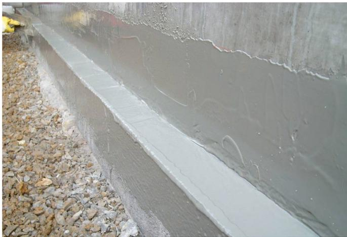
This data sheet is specifically for the application of Newton FlexProof-X1 to construction joints to concrete earth retained structures. For other uses of the product, please refer to the following Newton Data Sheets:
