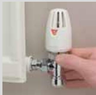
**4.** Remove manual shut off cap and store safely. With the sensor head set to the maximum setting (number 5) position the head so that the setting window can be viewed. Hand tighten the securing ring to fix the head in position.
