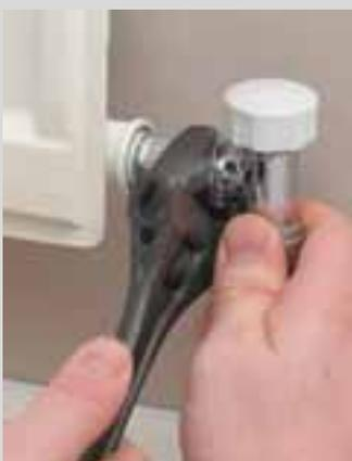
**3.** Connect the valve body to the tail, ensuring that the compression ring is seated centrally and that the tube makes firm contact with the tube stop in the valve body. Tighten nut, first using your fingers and then finish it by giving it a 3/4 to 1 turn with a high quality open ended or adjustable spanner.
