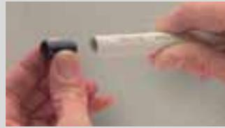
marks, ensuring there are no score marks on the pipe. Insert the correctly sized T66 pipe support liner from the Tectite accessories range fully into the pipe.
