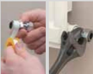
**2.** Apply a suitable PTFE based compound or PTFE tape to the threaded end of the tail. Screw 1/2" BSP tail into radiator and tighten using a high quality open ended or adjustable spanner.
