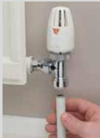
**5.** Push the tube/pipe firmly with a slight twisting action until it reaches the tube stop with a positive "click".
