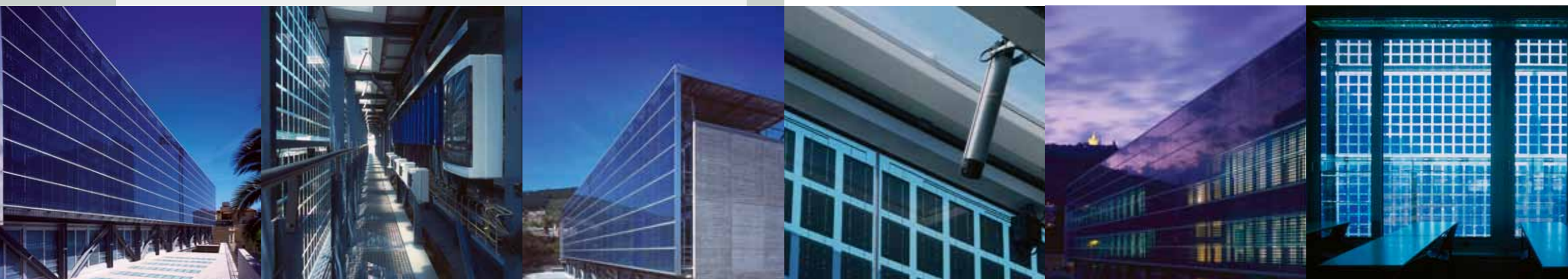
Curtain wall with photovoltaic panels - La Salle - Barcelona, Spain (Architect : Robert y Esteve Terradas Muntañola)
