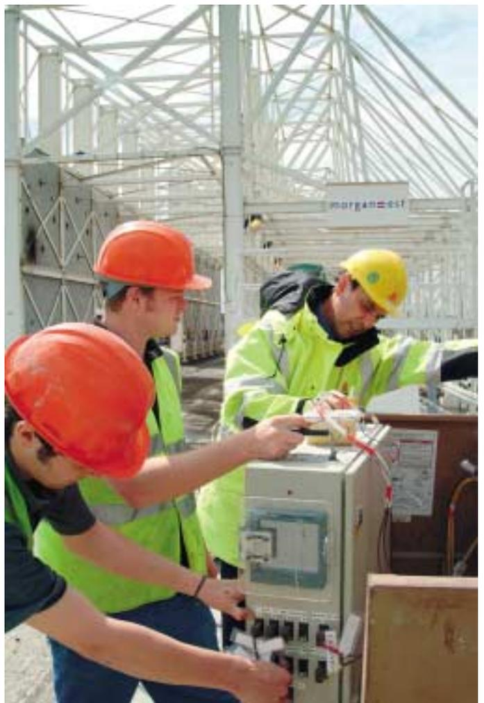
Connecting the Thermocouples to the Rapid Cure System monitor
