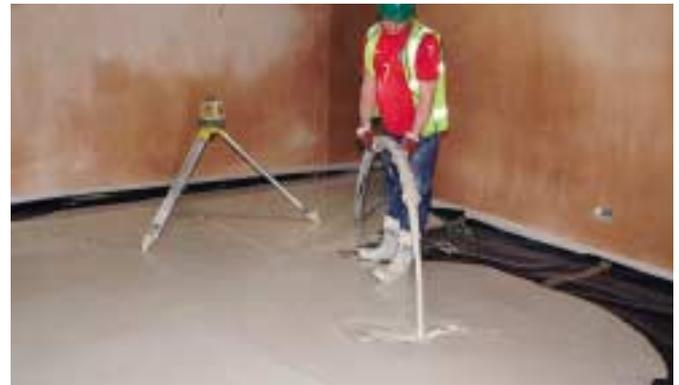
**Sika® SureFlow** being placed by pump to the required location
