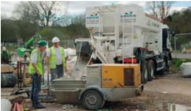
**Sika® SureFlow** being supplied using volumetric truck discharging into pump. minimal waste, optimised delivery quantities
