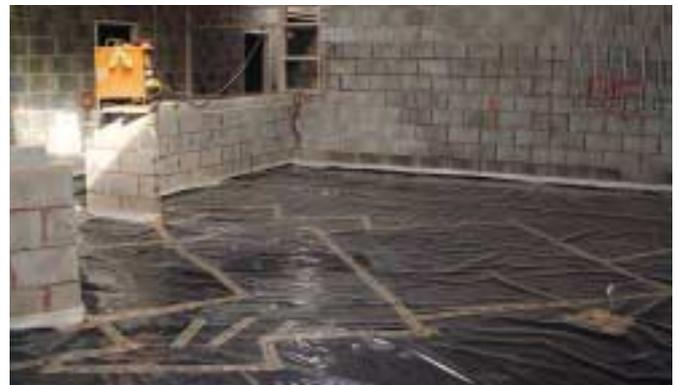
Prepared area with dpm and compression strip around the perimeter
