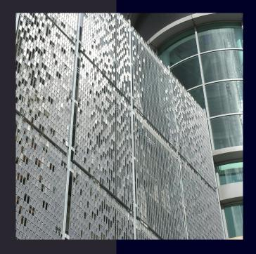
The STEREO-KINETIC® Wall façade was mounted on an independent steel frame which was bolted back to the existing structural steelwork.
