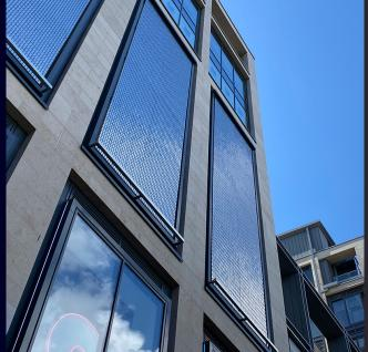
It was considered important that an art installation should form part of the facade, set within three recessed bays which had been constructed for this purpose.
