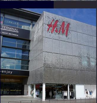
The stainless steel tiles of the STEREO-KINETIC® Wall panels were applied in a speckled pattern at second floor level to allow the passage of natural daylight through the underlying window openings.
