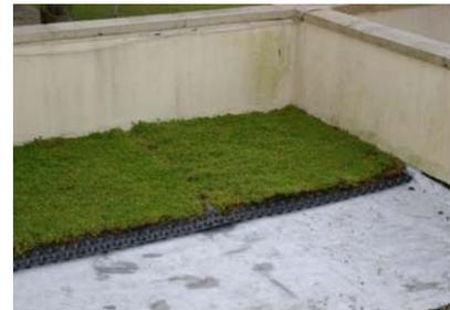
Each section has an overlap of Pro-drain 20P, so the egg-box shaped cells from one module can be fitted beneath the substrate of the next to achieve a secure and seamless fit together. No fixings are needed to go through into the deck, creating less disturbance to the waterproofing.
