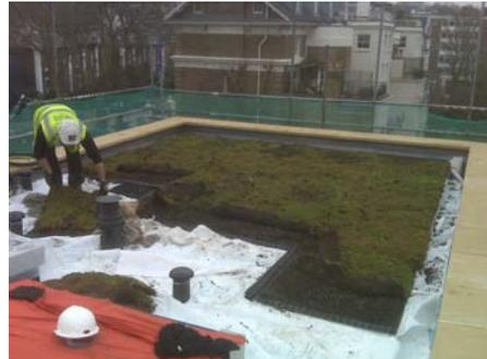
Each module is an established instant sedum roof system in itself, so when all trays are installed, the roof is finished. This cuts down on mess around site and the amount of space required to install the roof. Also, because these plants are fully established, they are less likely to be “shocked” once installed onto the roof and more likely to thrive quickly.
