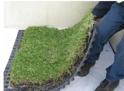
Installation couldn't be simpler. Just protect the waterproofing, lay the bottom layer of geotextile filter fabric and place the module into position on top.
