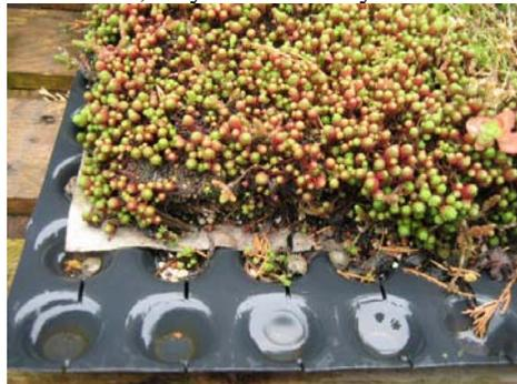
The build-up is the same as with the component green roof, each tray holding the Pro-drain 20P drainage sheeting, geotextile filter layer, approximately 70mm of aggregate based substrate and a sedum blanket.
