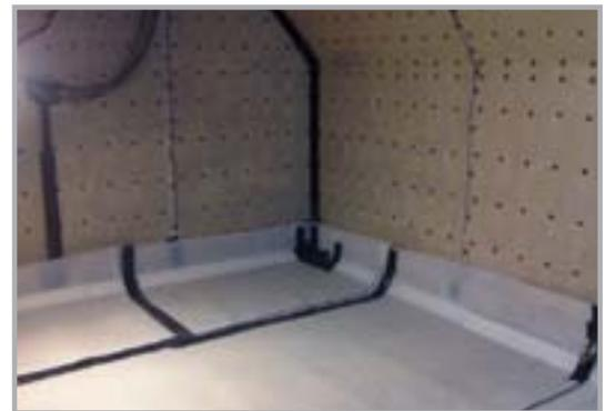
*The cavity drain option is recommended as it is fully maintainable and repairable*
