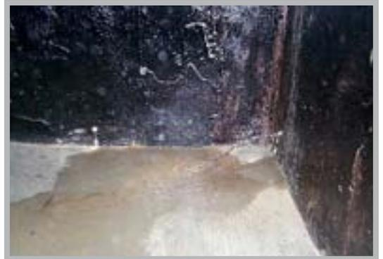
*Here bitumen paint has been applied as the tanking solution, and it has clearly failed*
