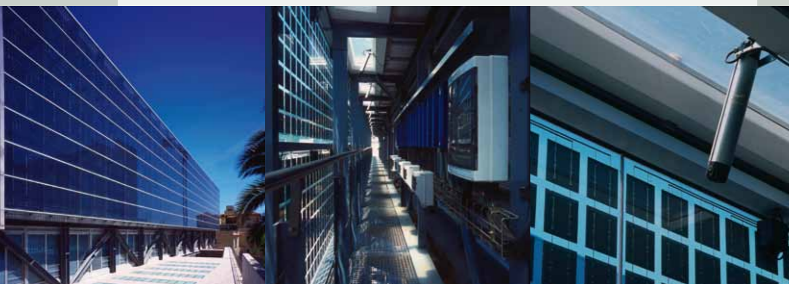
Curtain wall with photovoltaic panels - La Salle - Barcelona, Spain (Architect : Robert y Esteve Terradas Muntañola)
