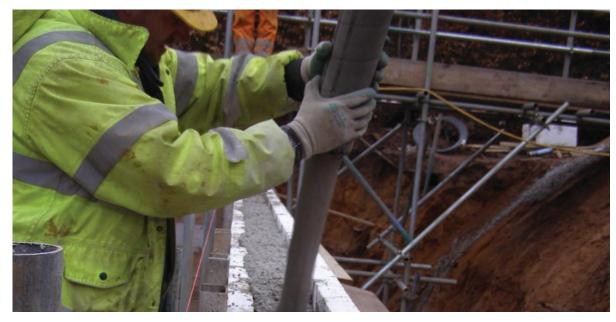
Widely used in the USA, Canada and Continental Europe, ICF (Insulating Concrete Formwork) is a relatively new UK building technique which involves a series of hollow expanded polystyrene blocks into which ICF-Crete® is poured. The system combines the inherent strength of concrete with the excellent thermal insulation properties of polystyrene to produce cost effective and durable structures.
