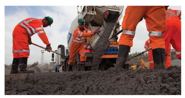
Emerald® is a range of concrete mixes that incorporate materials that are locally sourced where possible including secondary, recycled and reprocessed aggregates in addition to Portland Cement substitutes. Emerald® provides specifiers and contractors a fit-for-purpose concrete solution that has a reduced impact on the environment.
