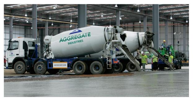
Extend™ is a range of low shrinkage concrete designed to reduce joint frequency for both flatwork and structural applications thus offering improved in-service performance and reduced construction costs.
