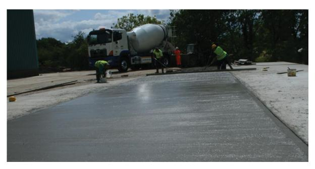
Highpave® is a range of fibre reinforced pavement grade ready-mixed concrete that reduce the errors associated with the use of conventional reinforcing methods.
