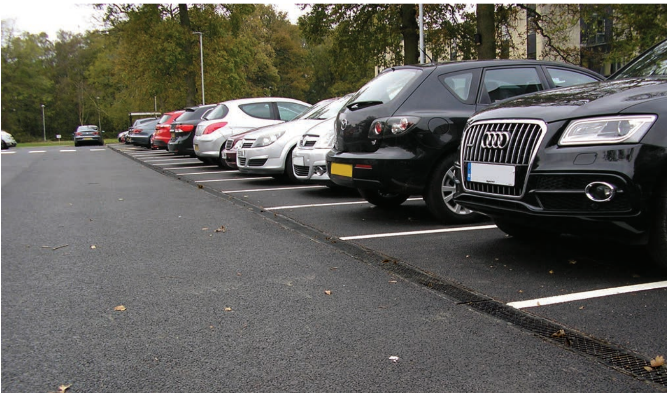
Fire Brigade Training Centre Car Park Moreton
