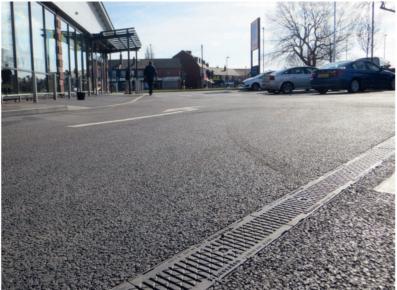
Car Park Middleton Leeds
