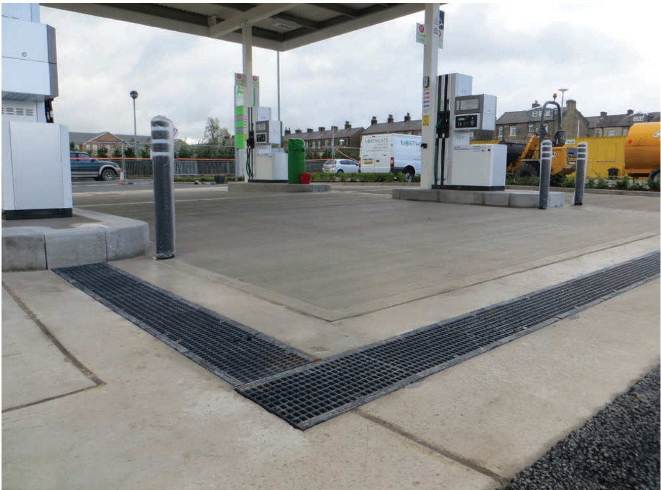
Petrol Filling Station , Dewsbury, Yorkshire
