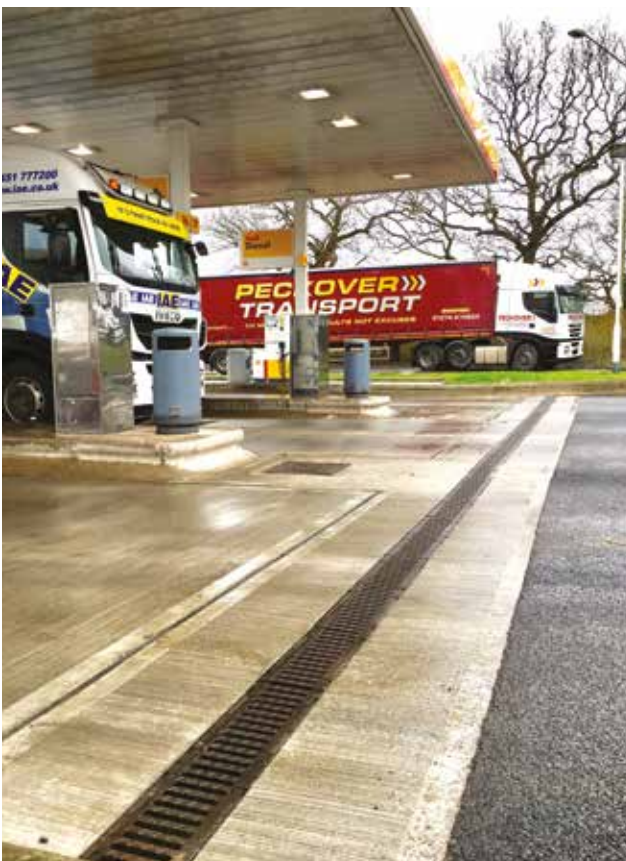
Charnock Richard Services HGV Refuelling Station
