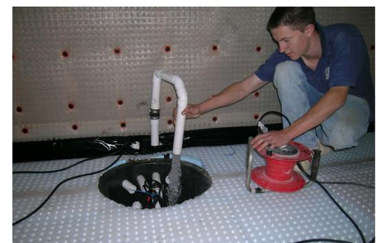
A Newton pump was installed with battery back-up protection in case of power failure
