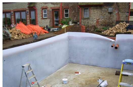
Newton 508 membrane applied to the walls of the new build basement
