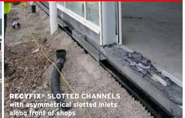
**RECYFIX® SLOTTED CHANNELS** with asymmetrical slotted inlets along front of shops
