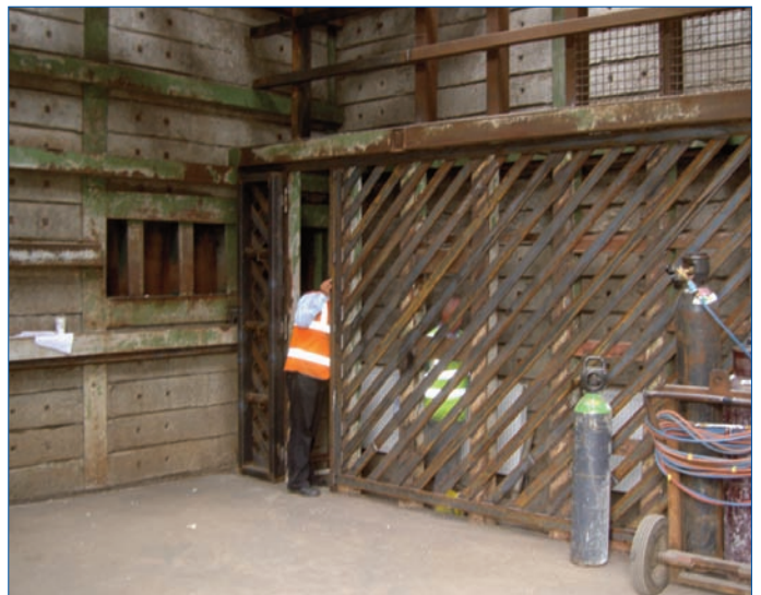
Inside view of the new elephant quarters showing safety corridor along one side of the stall, for keepers access
