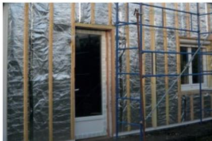
The quick and easy installation of 'all in one' Permafol offers a considerable labour saving against the multiple and complicated installation when cutting and fitting rigid and multi component products.
