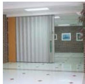
Wal-Mart Stores, the world's largest retailer and number four on the Fortune 500 list of US companies, recently installed the Won-Door FireGuard™ assembly in its new prototype retail outlets. Spanning 8' openings in one hour fire rated construction, they provide egress from the retail space to the stock room area.
