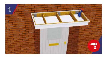
With canopy base in the desired position use a 10mm drill bit, drill through the rear structural timber rail into wall structure at a maximum of 450mm centres, to suit the StormFix 120 Fixing. The centre hole of the MS steel brackets can be used if appropriate.
