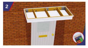
Insert StormFix Blue Frame Fixing sleeve 120 into the drilled holes. Once the StormFix Blue Fixing Sleeves have been inserted into the holes, fully screw the StormFix 120 fixings into the sleeves.
