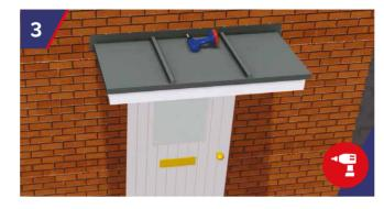
The roof unit is positioned onto the base unit. Using a 10mm drill bit, drill through the GRP upstand into wall structure at a maximum of 450mm centres, to suit the StormFix 80 Fixing.
