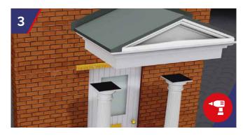
The Portico is placed on the columns, and the tops of the columns are screw fixed to the soffit of the portico. The soffit is screw fixed to the wall plate at 450m centres.
