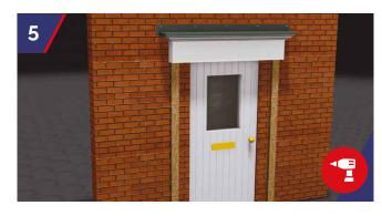
Once the StormFix Blue Fixing Sleeves have been inserted into the holes, fully screw the StormFix 80 fixings into the sleeves.
