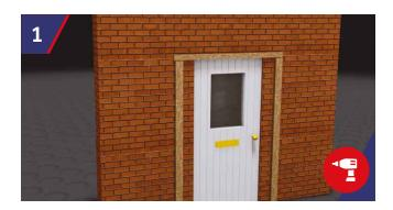
Contractor to fix timber frame securely to wall, by others on site, to suit the size of the GRP door surround.
