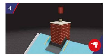
Insert tiling battens under the SmartStack gutter and simultaneously screw fix the GRP gutter and the tiling batten down onto the plywood using the screws supplied through all of the factory drilled holes. Unscrew lifting eye within SmartStack chimney pot and screw on SmartStack chimney pot onto threaded bolt.
