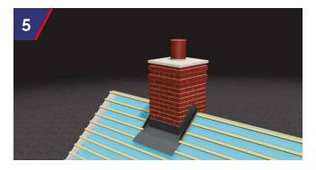
Batten out the roof. Lay a lead support fillet at the base of the chimney to ensure the lead is fully supported and on a continuous downward fall.
