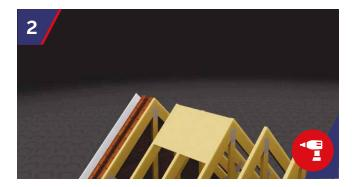
Screw fix the plywood panels to the noggins at a maximum 150mm centres and with minimum of 8 screws. It is imperative the plywood is securely fixed as the plywood will act as the main fixing point for the chimney.
