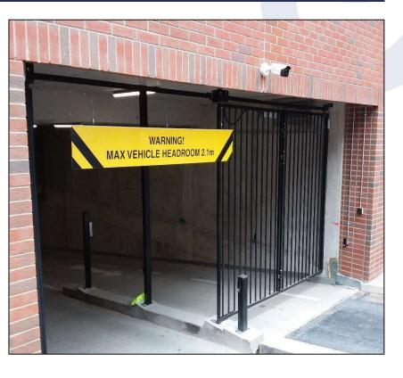
Disconnection for emergency manual operation is provided in the event of power failure.
