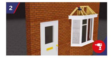
Using a 10mm drill bit, drill through the structural timber beam into wall structure at a maximum of 450mm centres, to suit the StormFix 120 Fixing.
