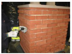
7. SECURE CHIMNEY TO SUPPORT FRAME Fix outer brick slip chimney to internal framework by screw fixing through mortar line directly into support frame. Fixings at 150mm vertical centres along each corner to each side. Minimum 10 fixings per side.
