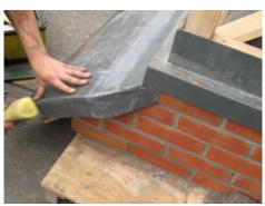
**10. DRESS LEAD AROUND PLINTH** Dress lead down over tiles immediately below dormer ensuring lead is on a continuous downward fall. Dress lead over edges of tiles to finish.
