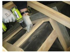
5. FIX INTERNAL SUPPORT FRAME Fix internal frame to plywood support using a minimum of 8 screws per side. (16 screws in total). Fixings to be around perimeter of support frame. Ensure frame is secure
