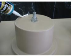
8. PREPARE FOR CHIMNEY POT Remove lifting ring and apply a bead of adhesive
