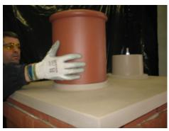
9. SECURE CHIMNEY POT Locate GRP pot screw into position. Seal around base of pot as appropriate
