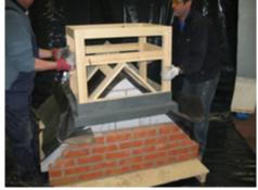
4. POSITION INTERNAL SUPPORT FRAME Position frame onto roof structure ensuring downstand to plinth box is tight to and cloaks over the external brickwork. Ensure internal frame rests fully onto roof structure with no movement
