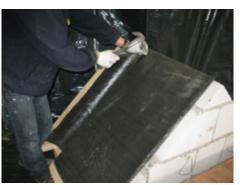
**3. APPLY ROOFING MEMBRANE** Fix 38 x 50 timber noggins to the side of each rafter. Apply roofing membrane to the whole of the roof structure as per standard roofing practice.
