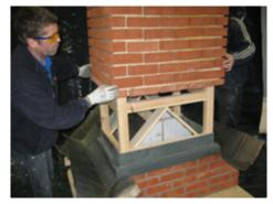
6. POSITION BRICK SLIP CHIMNEY Carefully lower the brick slip chimney over the secure support frame until it rests fully onto plinth box.
