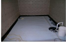
Newton 508 Mesh cavity drain membrane was fitted to the walls and vaulted ceiling, and Newton 508 was loose laid to the slab and taped to form a vapour seal
