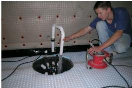
A Newton pump was installed with battery back-up protection in case of power failure
