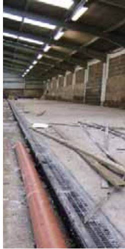
The GUGI® mesh grating which has a Class B125 loading, allows quick water ingress during wash down
