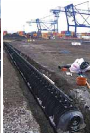
RECYFIX® HICAP® High Capacity drainage channel
