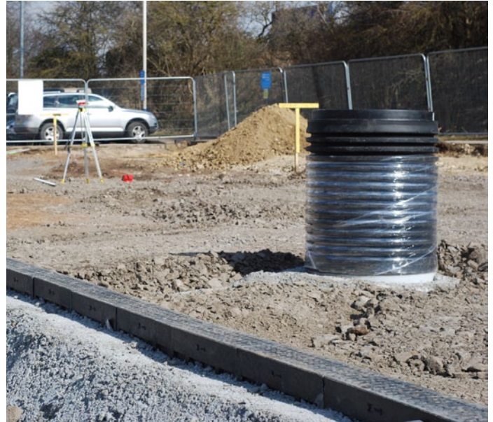
ACO Q-Ceptor and ACO ParkDrain during installation.
