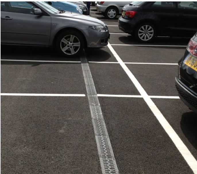
ACO ParkDrain efficiently collects surface water run off.
