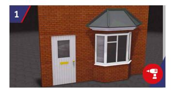
The GRP bay window roof is placed centrally onto the bay window. The bay window roof soffit should be level and large bay window roofs should have support props prior to fixing.
