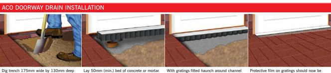
Dig trench 175mm wide by 130mm deep for channel. If draining to a soakaway, remove cut outs in end caps and fit to channel or, if connecting to underground pipework, knockout a preformed outlet at the required position in the base of the channel unit and fit the outlet connector.
