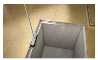
**Step 9:** Once the final floor or pavement has been fully installed, remove any excess adhesive or grout from around the cover and frame. Open the cover with the lifting/locking keys provided. Clean all surfaces and ensure the seating areas of the cover, rubber seals and hinges where fitted are free from debris. Lubricate all seals and hinges with a suitable silicone grease.
