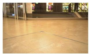
**Step 10:** Close/refit the cover and check that there is an even gap between the cover and frame. Insert all locking screws and hand tighten to securely lock the cover. Refit all locking screws dust caps. Once all installation materials have fully cured, the access cover is now ready for use and service loads. Retain all spare parts, the installation and maintenance booklet and lifting/locking keys for future use.
