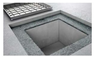
Step 5: Lay a mortar bed of minimum 40mm thickness all round the shaft opening covering the full width of the frame. Minimum mortar class M6 to BS EN 998-2:2016. For ASSIST covers only level the cover and frame centrally over the shaft and shutter internal clear opening. Use minimum grade C35/45 concrete to BS EN 206:2013 to anchor and bed the ASSIST frame. Allow concrete to sufficiently harden before removing shutter. Ensure the ASSIST frame is fully supported by the concrete bed with no voids.
