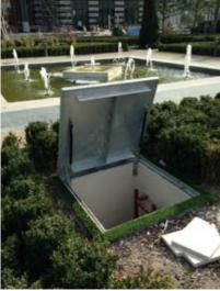
With a comprehensive range of standard clear opening sizes from 200 to 1200mm, ACO floor access cover can be supplied either as single units or for ducting and multi span applications. Manual lift or gas spring assisted versions are also available to suit the intended method of opening, frequency and ease of operation.
