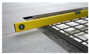
**Step 6:** Bend out steel anchors horizontally. Bed and level the access cover and frame centrally over the shaft opening. When tapping down to level use a piece of wood to protect metal surfaces. Ensure the frame is fully supported by the mortar bed with no voids. Allow mortar to sufficiently harden. Insert spacers between the frame and cover to maintain an even gap.
