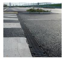
To support a wide variety of catchment depths, hydraulic capacities and applications, the system is available in four channel widths and is offered in constant and sloping depths for optimum performance and system design.
