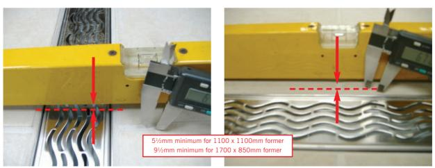
Figure B. Checking falls to channel – both ways
