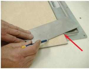
Figure A. Cutting tiles to visible channel corner - allow for grout width
