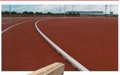
Available as straight and radius units with an anchorage groove for track surfacing on one side, both sides, or with no groove.
