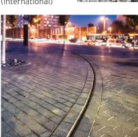
\*The A-symmetric slotted cover can be used along building facades, walls and landscape features at ground level.
