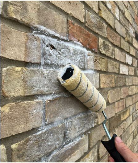
5.1.2 Roll applied Passivhaus Brick Seal
