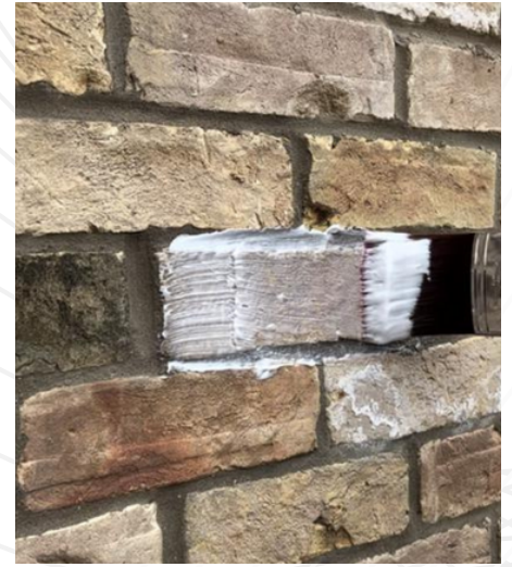
5.1.4 Brush applied Passivhaus Brick Seal
